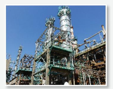
• Naptha Hydrotreating Unit, 33,400bpd, Built 1969, Upgraded in 1991 & 2010, Licensor is UOP
